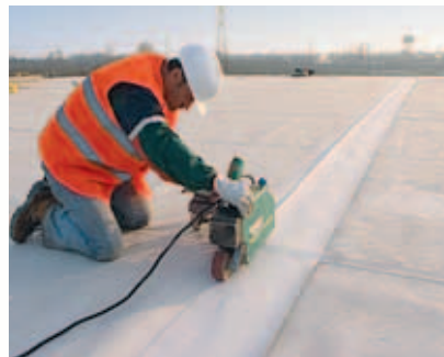
Soldadura de la junta / Overlap Welding
